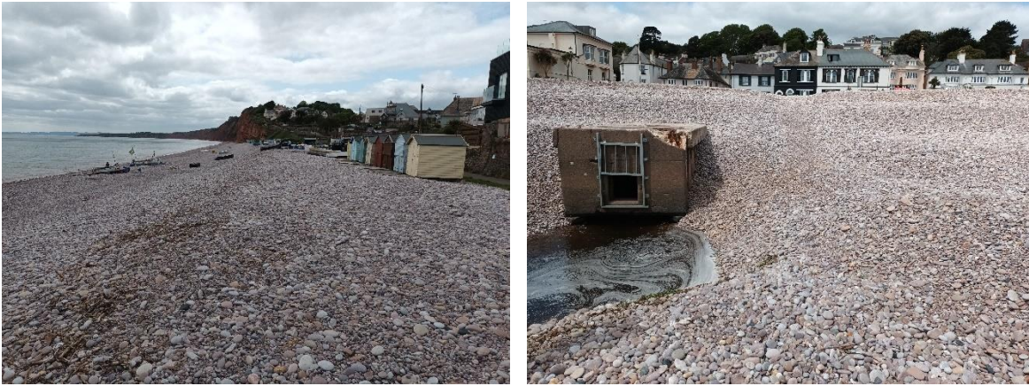
Figure 4: View westwards along the beach from within policy unit 6a41 (left) and view north of one of the outfalls that regularly gets blocked by shingle, posing an upstream flood risk (May 2024).
